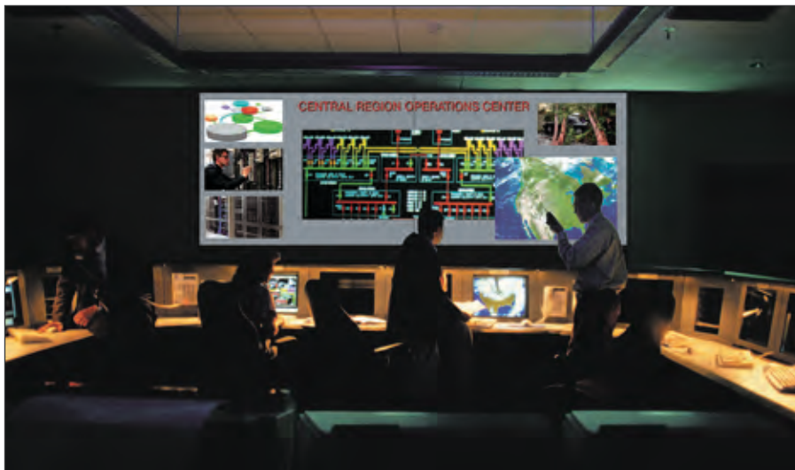
Network operations centers often use a fully digital signal distribution architecture to deliver high quality, high resolution images.
